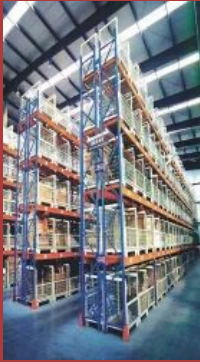
Palletized cold storage
