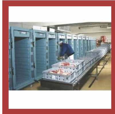
Meat Cold Storage Plant
