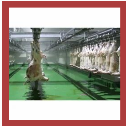
Meat Processing plant
