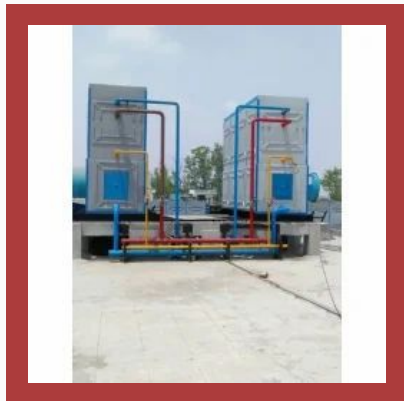
Industrial Evaporative Condenser
