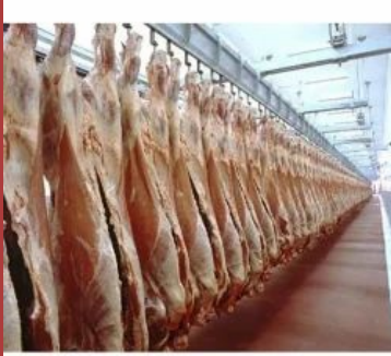
Chiller Meat Freezer
